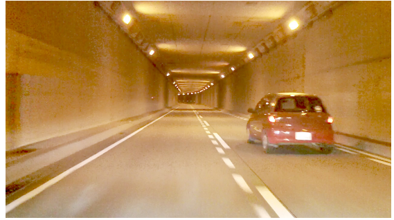
(b) A tunnel.
